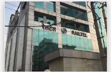
Railtel DC Gurgaon
