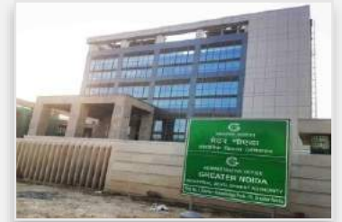
Noida Authority PCC Electrification
